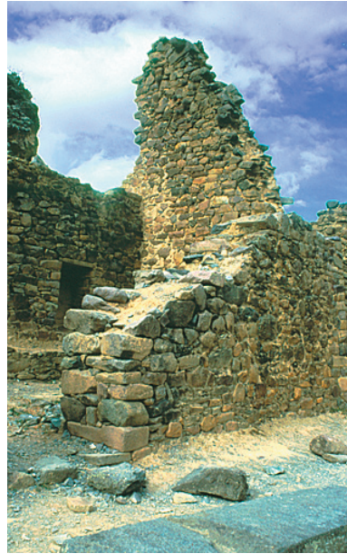
Much of the ancient Inca fortress structure at Ollantaytambo remains intact today, although the temple shrine was never completed. Various granites, limestone, basalt, and even sandstone can be found at the ruin site.
